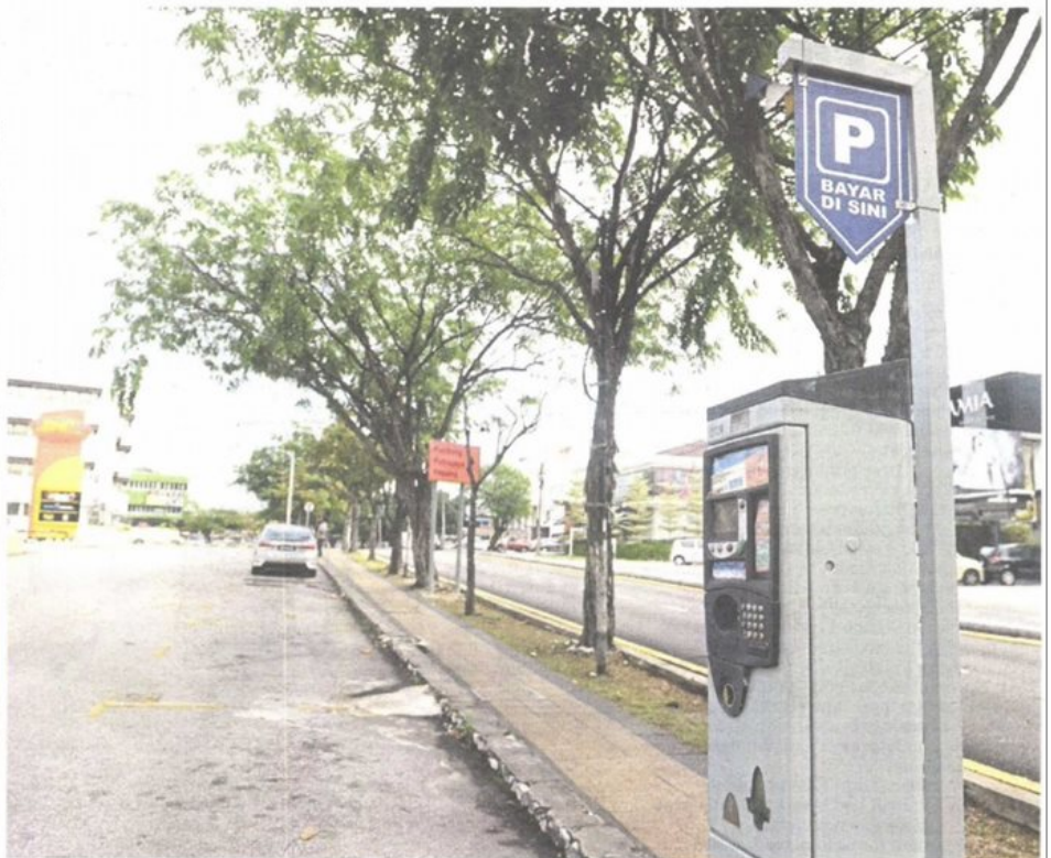
There are numerous complaints over the faulty parking machines in Petaling Jaya. A reader said he found faulty meters in PJ New Town, PJ Old Town and Jalan Gasing.
