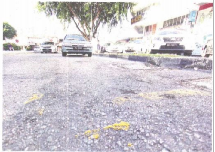
Yeo says the parking boxes must also be clearly painted.
